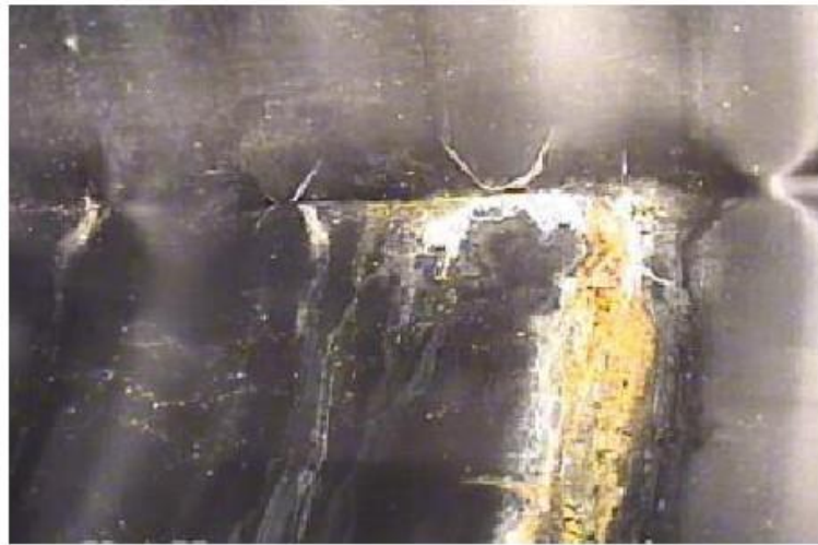
Wall Crushing/Cracks
