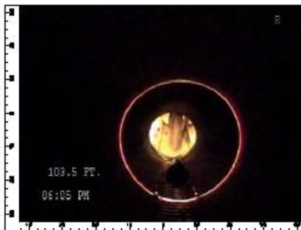
Pipe round at 103.5 ft.
