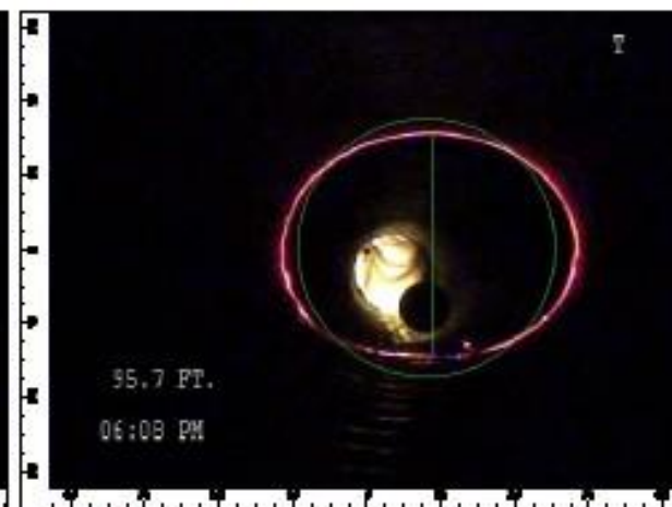
Pipe deflected approximately 14.6%.
